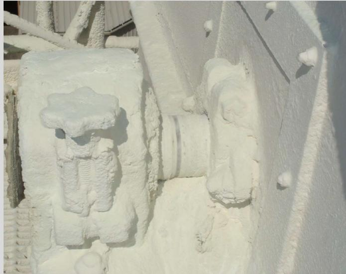
**Before:** Lime dust leaking onto adjacent pillow block bearing and surrounding area
